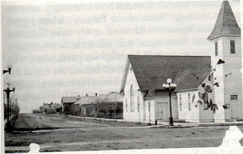
Trinity Methodist Church, 1903, extended in 1907, became the United Church of Estevan in 1921 and St. Paul's United Church in 1931 and was extended again in 1949.
